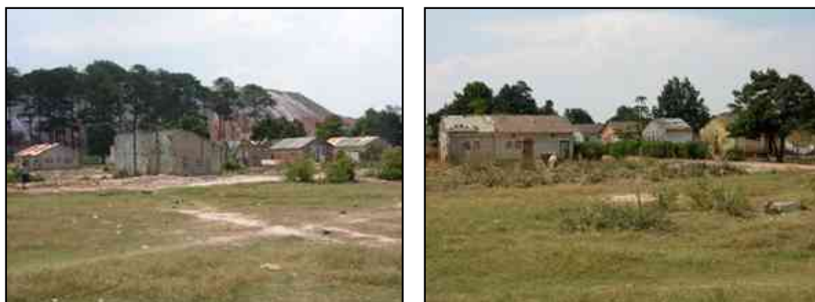
Picture 40: Musonoi: in some parts of the township, mainly the parts which were supposed to be relocated, houses are in a very poor state
