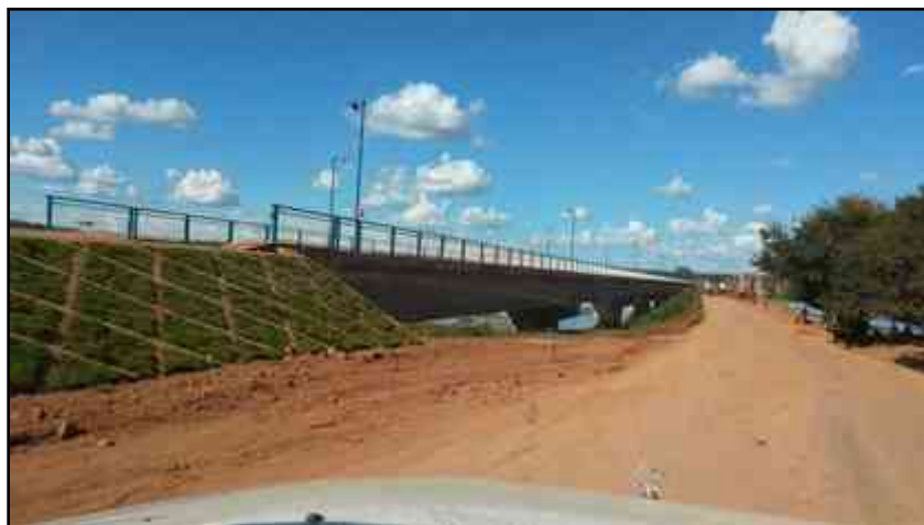
Picture 31: The new Lualaba bridge
